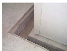
Excavation sample Dettaglio scavo
